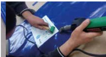
*Carefully walk over the entire contact surface with the roller, especially over the joints.*
